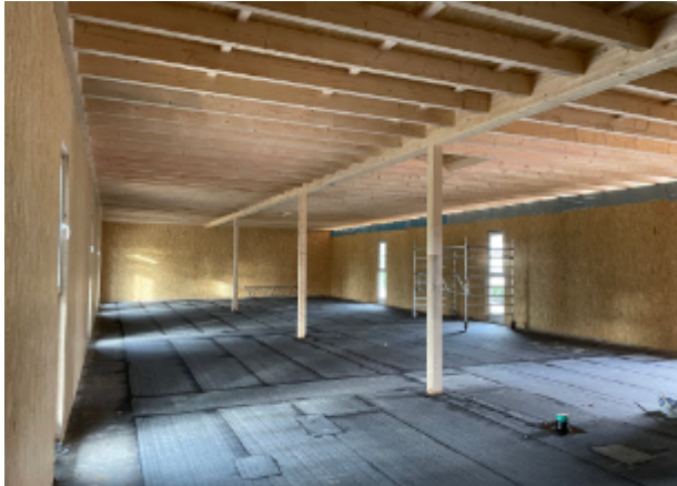
Caddy-Halle, innen Rohbau
